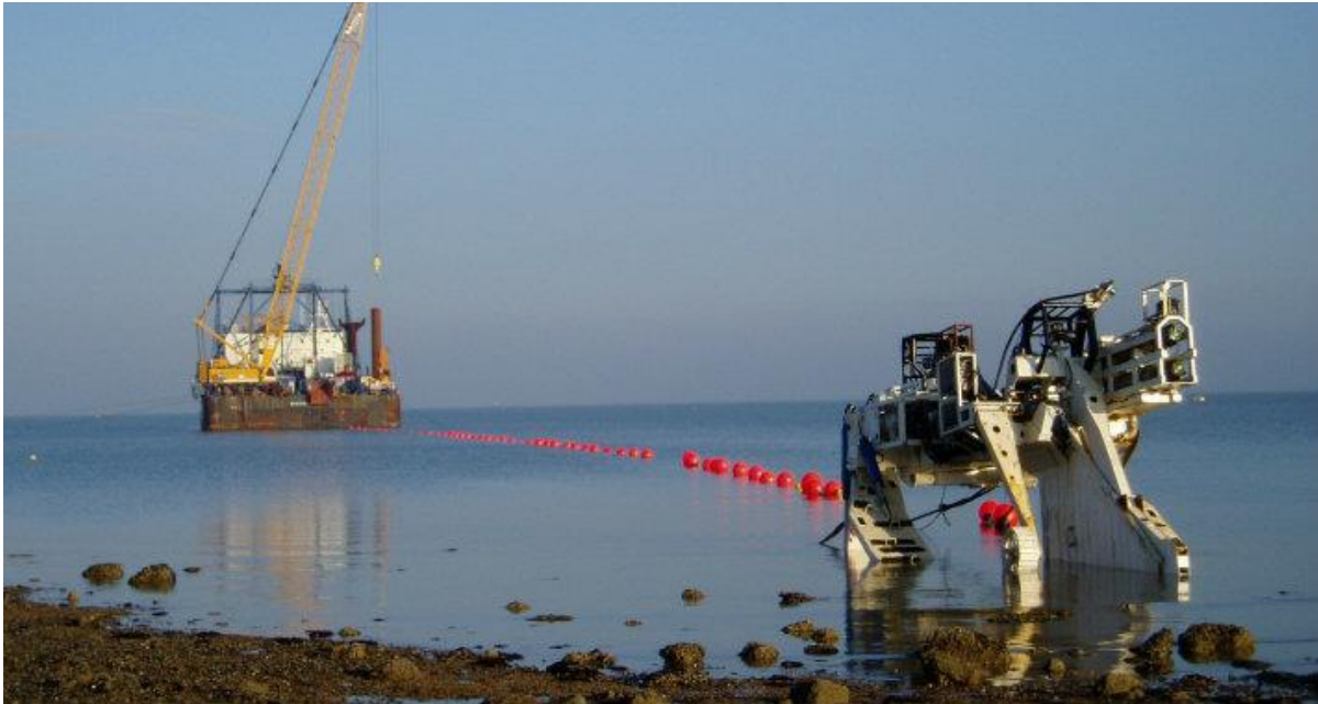
Figure 19: Global Marine's Hi-Plough
